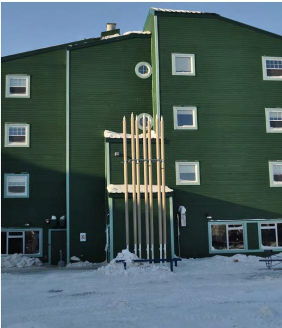
**Figure F16.** Example of thermosyphons, a foundation system that requires a significant amount of expertise to design, install, maintain and monitor (CSA, 2014).
