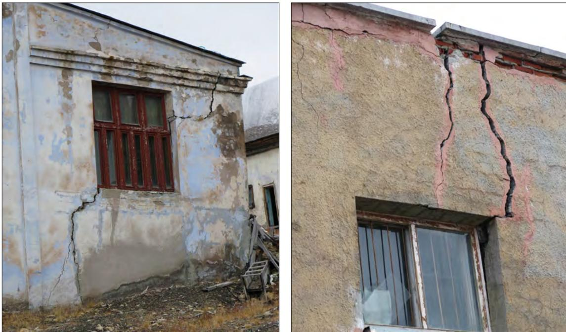
**Figure F3.** Examples of unmaintained buildings in Pyramiden, Svalbard, displaying cracks and uneven settlement in response to permafrost thaw.
