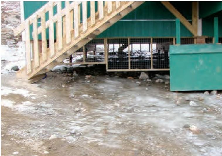
**Figure F18.** Example of water ponding around a foundation built on permafrost (Government of Nunavut, 2013). Water ponding can have a negative impact on permafrost thermal regimes.
