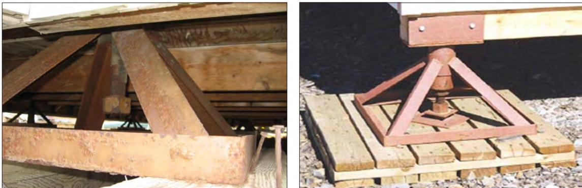
**Figure F11.** Examples of adjustable-jack foundations from Gravel (2012) and CSA (2010).
