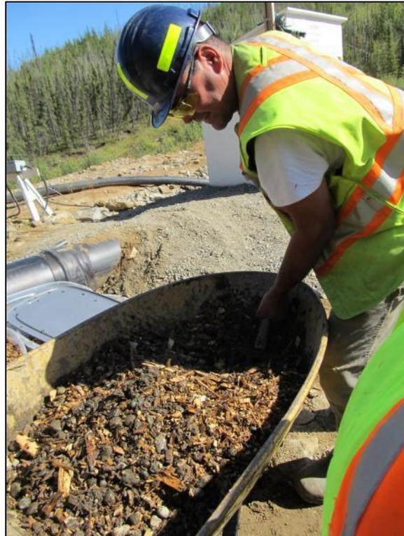
**Figure 4.** Bioreactors substrate mixture preparation.
