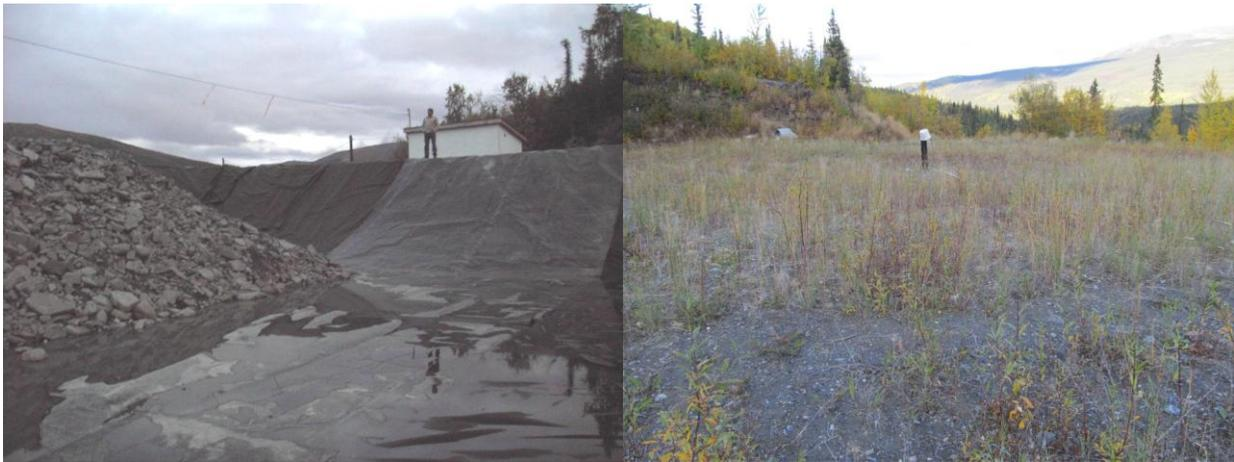
**Figure 7: Bellekeno pilot bioreactor under construction in 2008 (left) and after 5 years (right) (Alexco, 2012, p. 6).**
