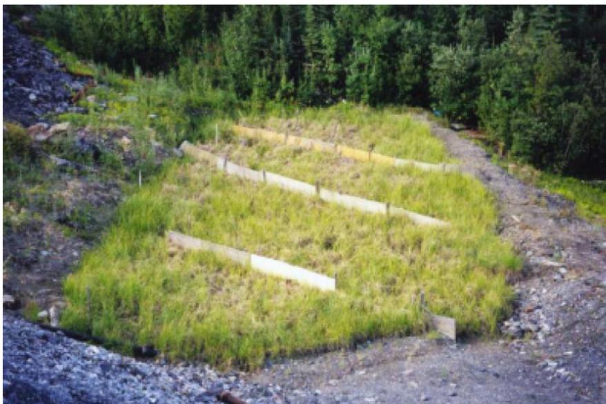
**Figure 6: CW at Galkeno 900 adit with plywood baffles to help distribute flow evenly (Burns, 2000, p.38).**
