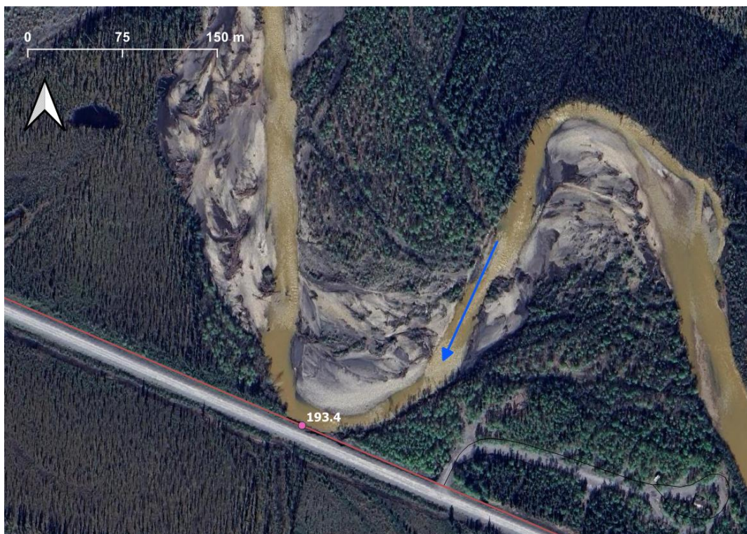
Figure 7. KM 193.4 of Dempster Highway. Separation distance = 0 m, risk rating = Very High, imagery date: June 4, 2023.
