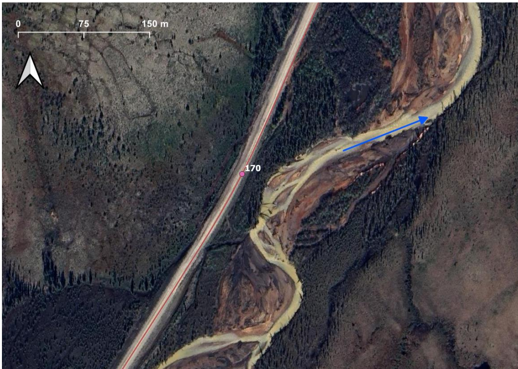
Figure 3. KM 170.0 of Dempster Highway. Separation distance = 25 m, risk rating = High, imagery date: June 4, 2023.
