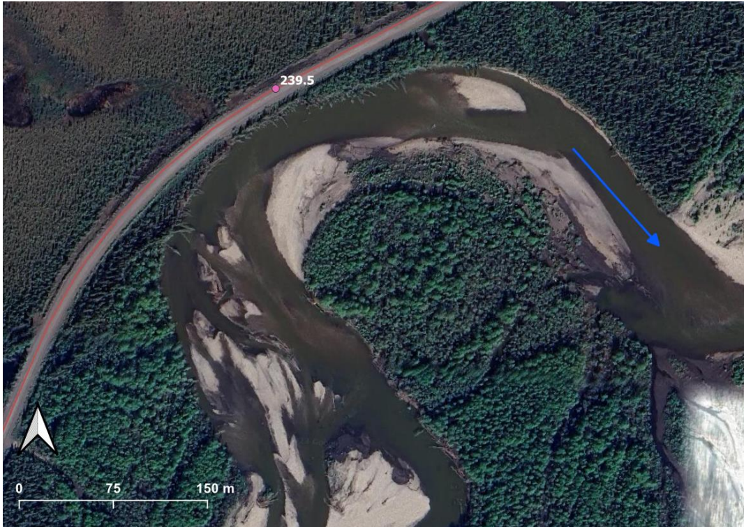
Figure 11. KM 239.5 of Dempster Highway. Separation distance = 6 m, risk rating = Very High, imagery date: June 7, 2023.
