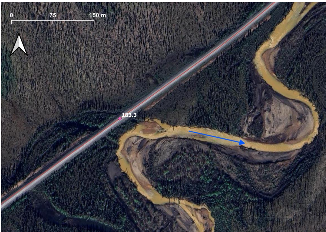
Figure 6. KM 183.3 of Dempster Highway. Separation distance = 18 m, risk rating = High, imagery date: June 4, 2023.
