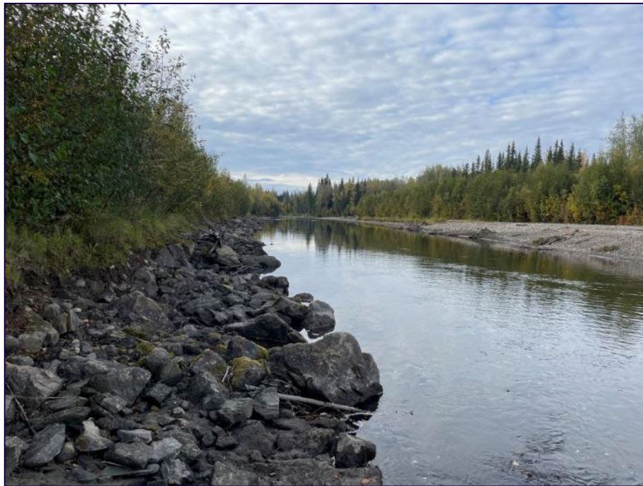
FIGURE 6.6. RIPRAP PLACED ALONG THE BANK OF KLONDIKE RIVER ADJACENT THE NORTH KLONDIKE HIGHWAY DOWNSTREAM OF KM 665.8.
