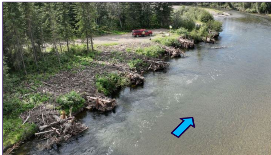
FIGURE 6.5. CONSTRUCTED WOOD ‘SPURS’ ALONG THE REGULATED MAYO RIVER THAT DEFLECT ENERGY AWAY FROM THE BANK (PHOTO CREDIT: ECOLOGICAL LOGISTICS AND RESEARCH LTD.).
