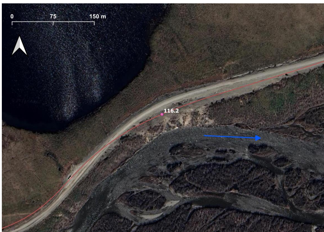
Figure 2. KM 116.2 of Dempster Highway. Separation distance = 16 m, risk rating = High, imagery date: June 2, 2023.
