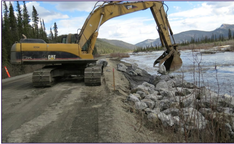
FIGURE 6.8. CAREFUL PLACEMENT OF RIPRAP ON AN EMBANKMENT USING SPECIALIZED EQUIPMENT LEADS TO BETTER LONG-TERM RESULTS (PHOTO CREDIT: HPW). NOTE THAT IN THIS PHOTO, THE RIPRAP IS CAREFULLY BEING PLACED ATOP GEOTEXTILE, WHICH CAN FORM A SLIP-SURFACE AND CONTRIBUTE TO REVETMENT FAILURE. A PROPERLY GRADED STRUCTURE WITH A SUBSTRATE MADE OF SAND AND GRAVEL REPRESENTS A SUITABLE ALTERNATIVE. LOCATION: DEMPSTER HIGHWAY KM 179.6.
