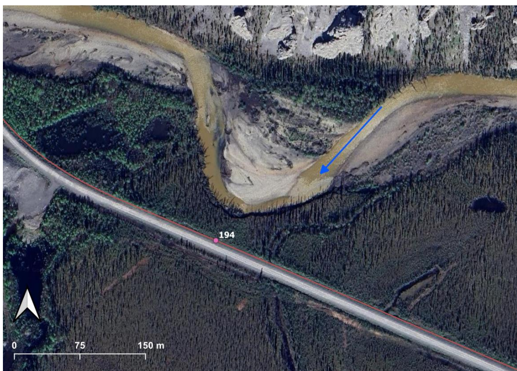
Figure 8. KM 194.0 of Dempster Highway. Separation distance = 28 m, risk rating = High, imagery date: June 4, 2023.
