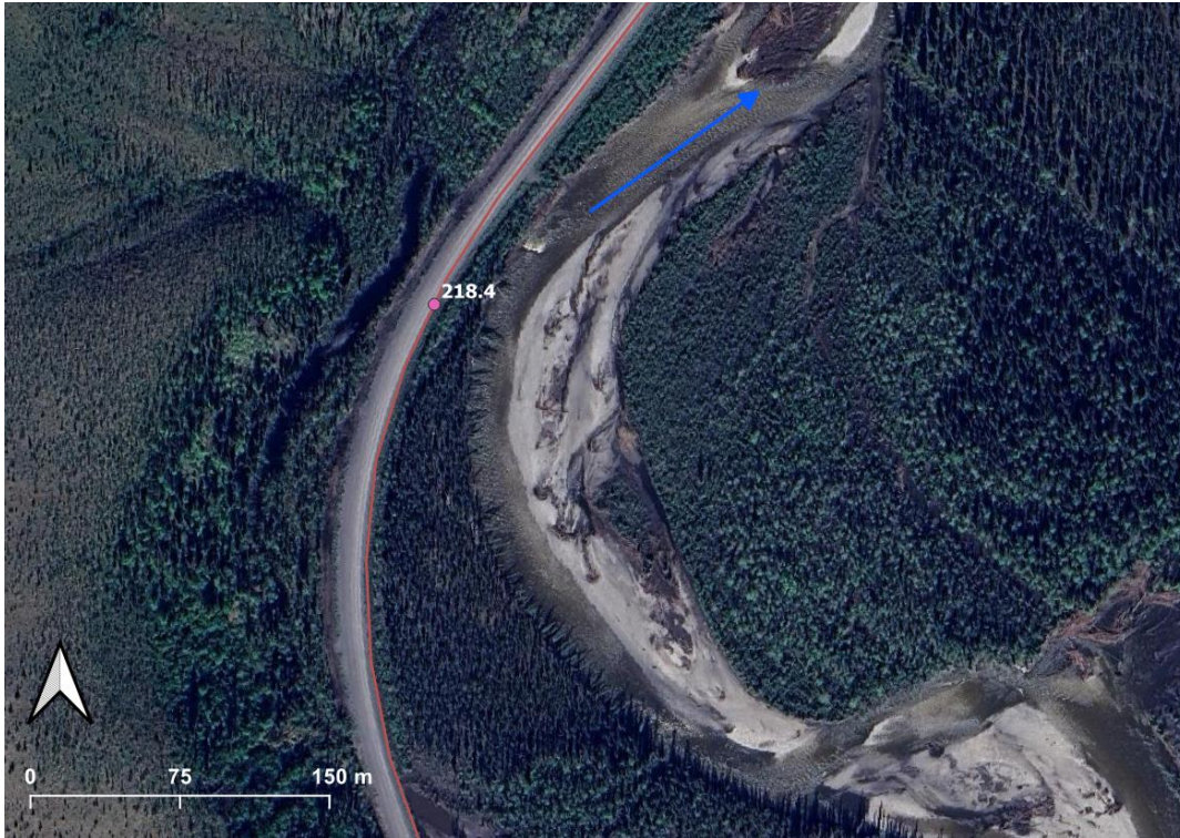
Figure 9. KM 218.4 of Dempster Highway. Separation distance = 13 m, risk rating = High, imagery date: June 4, 2023.
