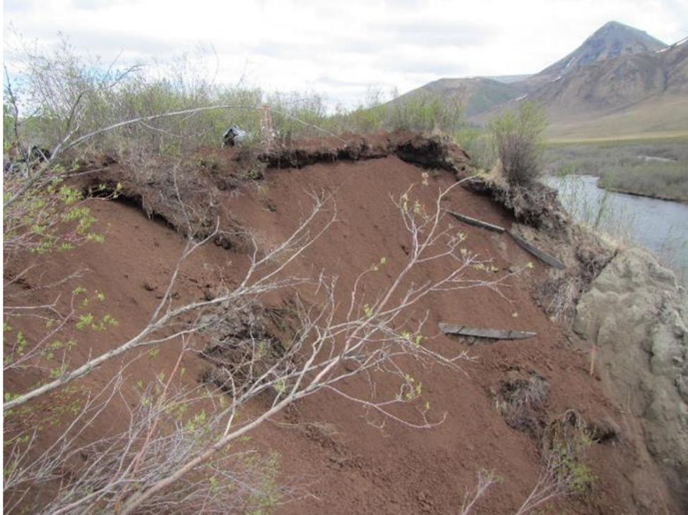
**Figure 39** Peat cover installed in September 2018 to the 2017 thaw slump.
