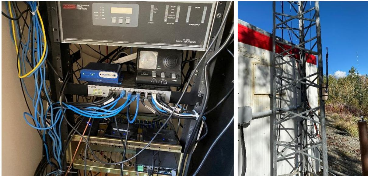
**Figure 118.** Multitech gateway installation. Left - Gateway (blue box) connected to the internet at local farm. Right - Gateway antenna communicating with LogR Systems ULOGC32 LoRa+ logger located 1060 m away.
