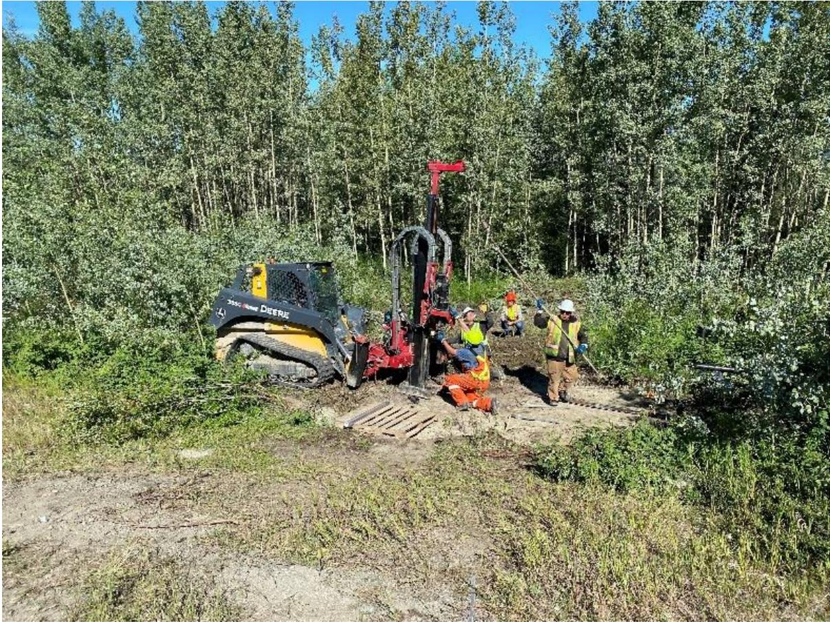
**Figure 98** Borehole drilling at Takhini RTS site using Direct Push Technology (DPT) system.
