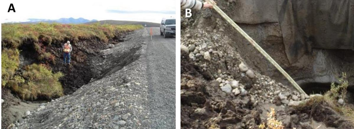
**Figure 35** Degradation observed in summer 2006 along the newly built embankment at km 116. A- thermal erosion along the left-hand side shoulder; B- water tunneling under the embankment along an ice-wedge.
