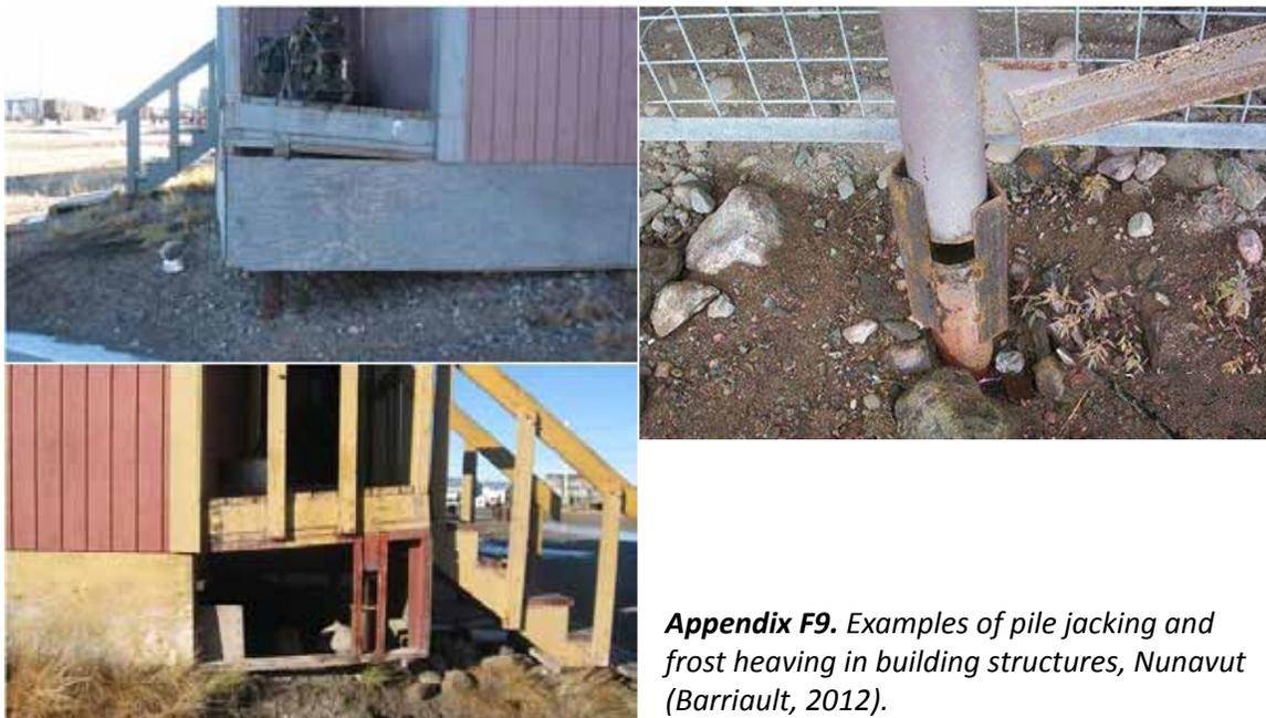
**Appendix F9.** Examples of pile jacking and frost heaving in building structures, Nunavut (Barriault, 2012).
