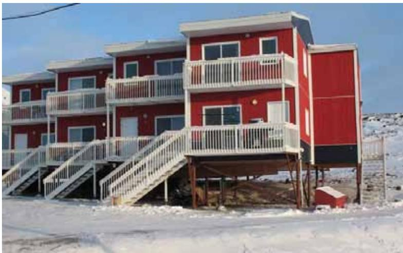
**Appendix F8.** Housing built on steel piles (Gravel, 2012).
