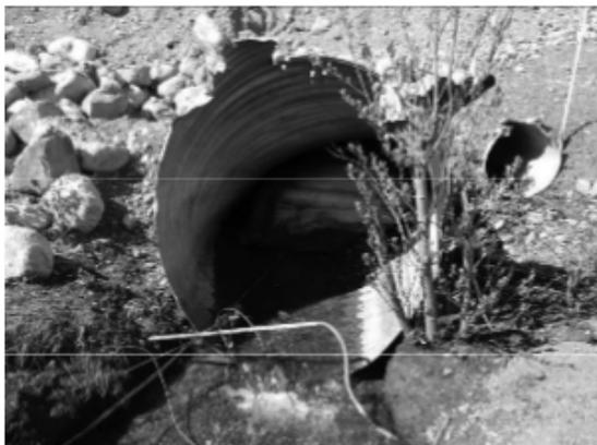
Figure 7. Culvert at km 32.5 (North Klondike River valley), filled with icing, May 2014. Photo by C.R. Burn.
