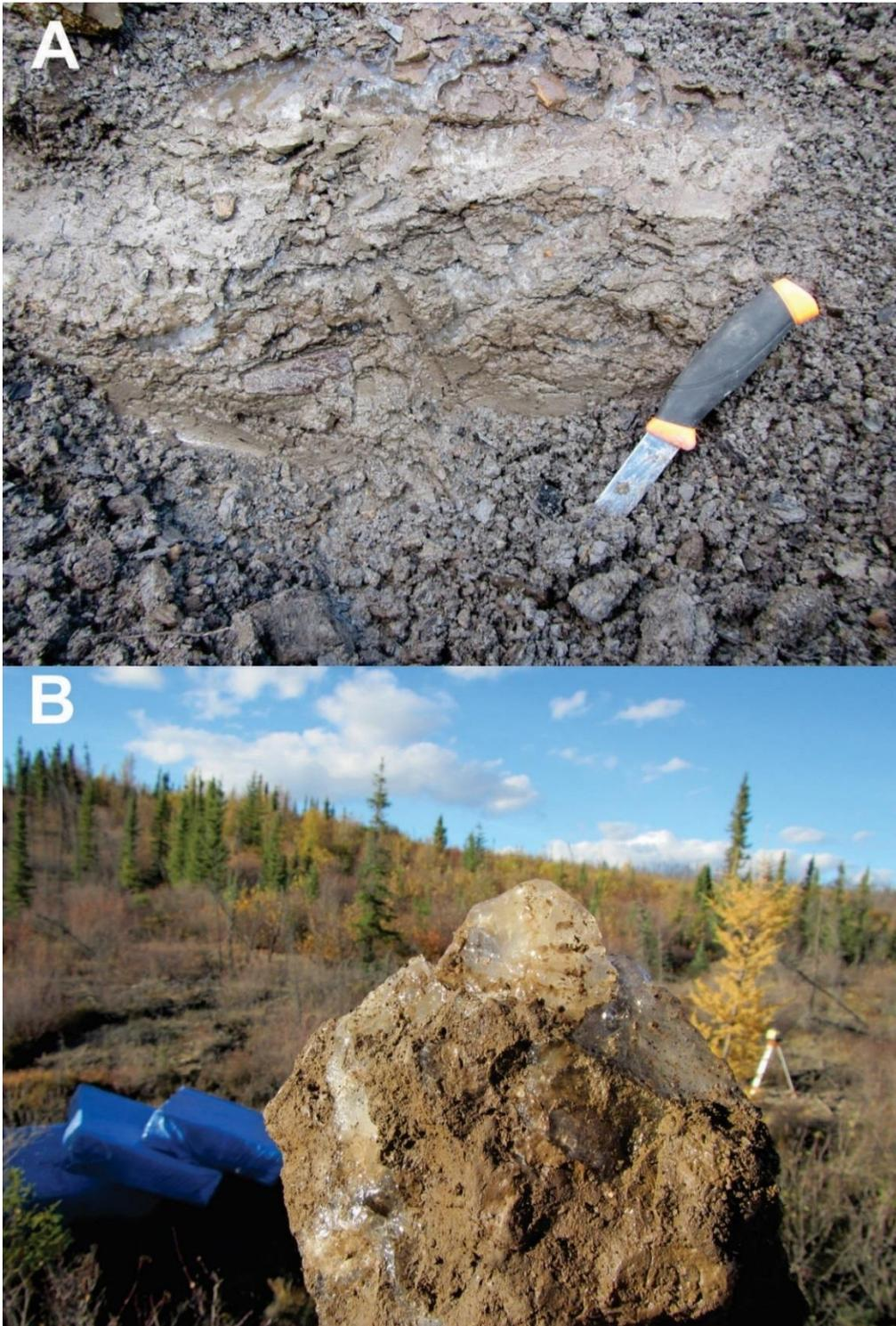
**Figure 3.10.4** Permafrost observed during culvert installation at site DH381. A- ice-rich fine grained soil excavated below the embankment; B- close-up of an ice-rich permafrost sample collected during the excavation works
