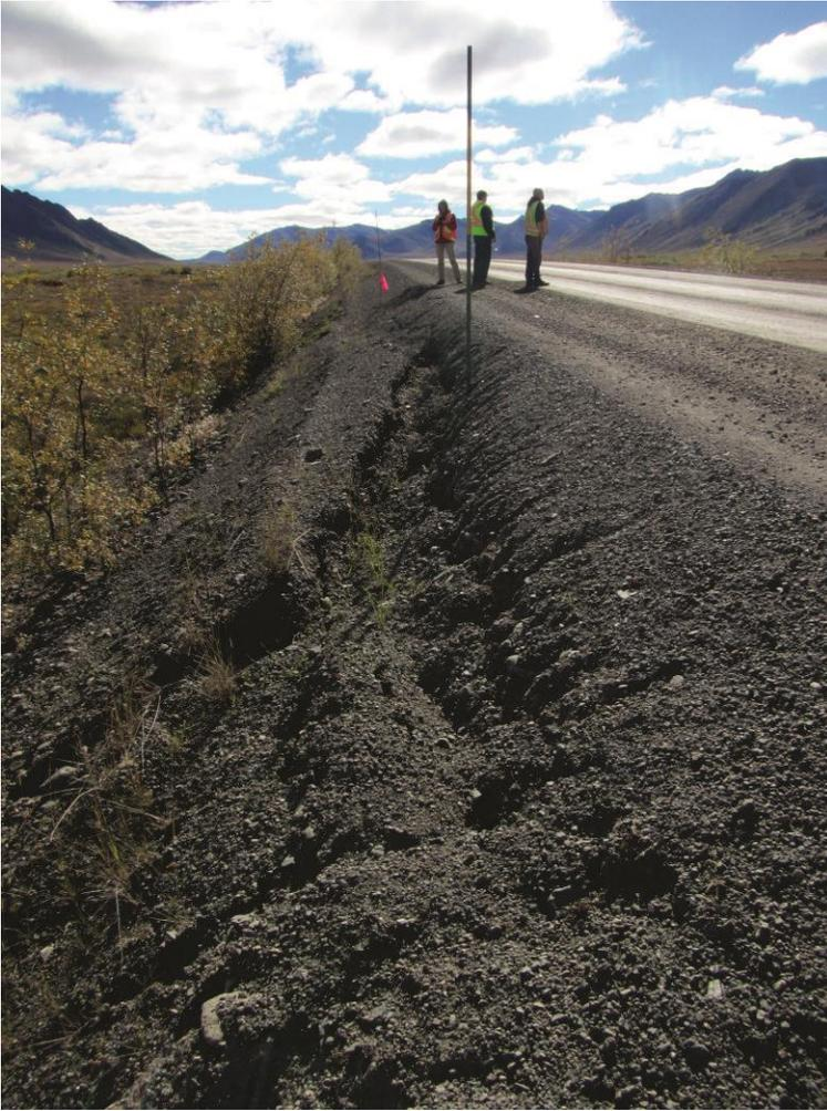
**Figure 3.2.1** 20m failure located on the RHS of the road at site DH95.
