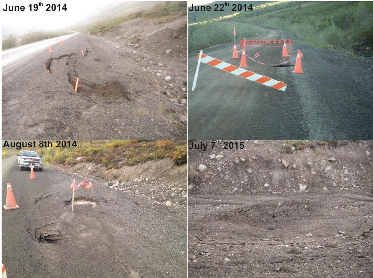
**Figure 3.1.1** Degradation observed at site DH82 in 2014 and 2015.
