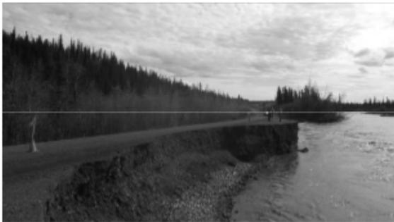
Figure 10. Wash out of the road by Ogilvie River at km 245, June 2013. Photo by S.N. Orban
