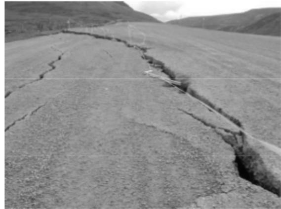
Figure 11. Thaw subsidence of the embankment at NT km 27, August 2011. Photo by C.R. Burn.
