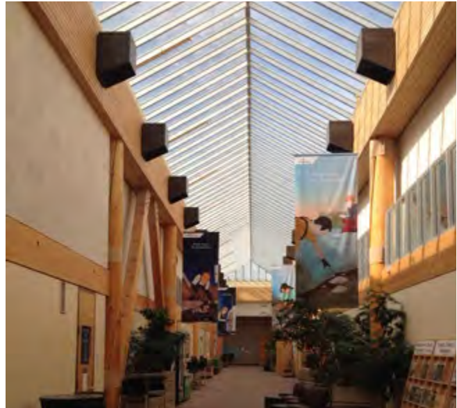
Figure 11 - Skylights provide daylight within the internal circulation networks of the a-, c-, and t-wings
