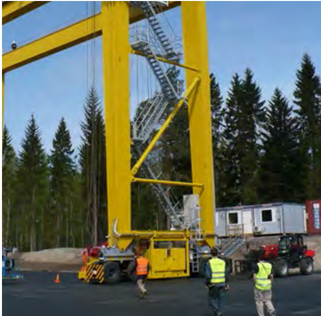
Access for Trucks and Machinery
