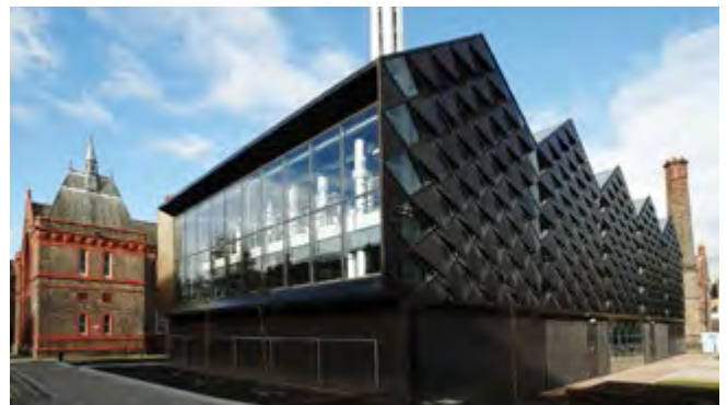
District Energy plant
